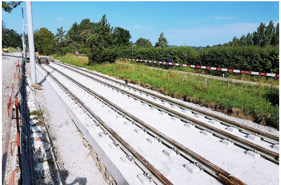
Abb. 7: Gleistragplatte System Rheda City.
